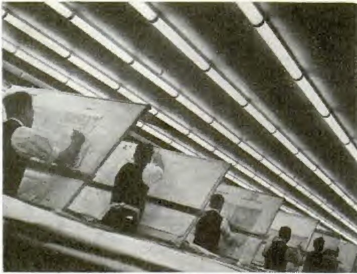
"Daylight" around the clock is supplied by one-third of a mile of fluorescent lamps in large drafting room of a Westinghouse plant.
